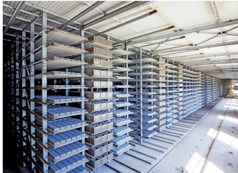
Well-coordinated and customised solutions: storage and retrieval logistics in the curing area
