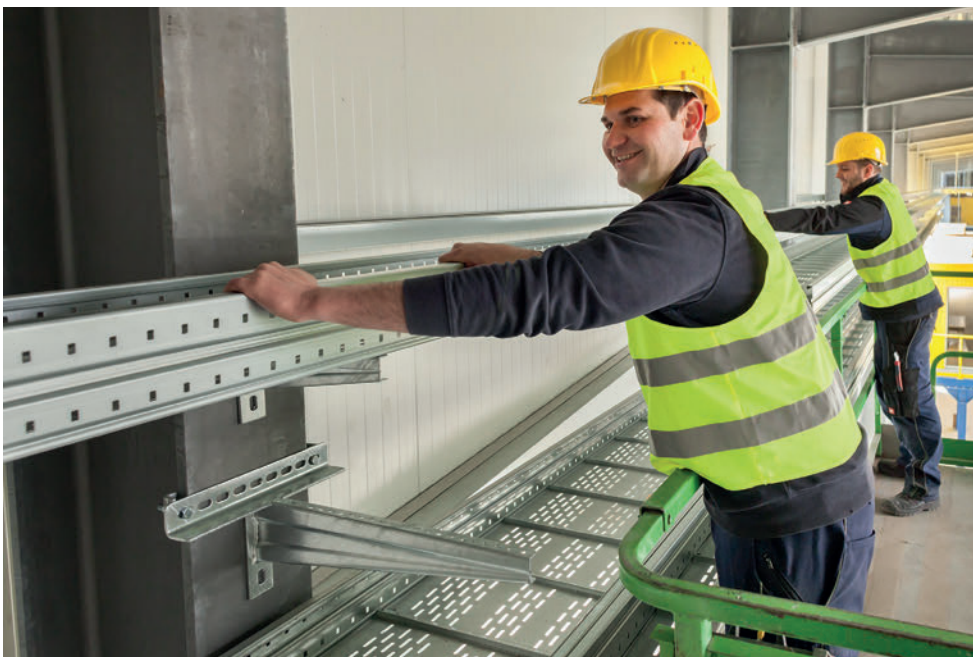
Professional and just-in-time: laying the new cables
