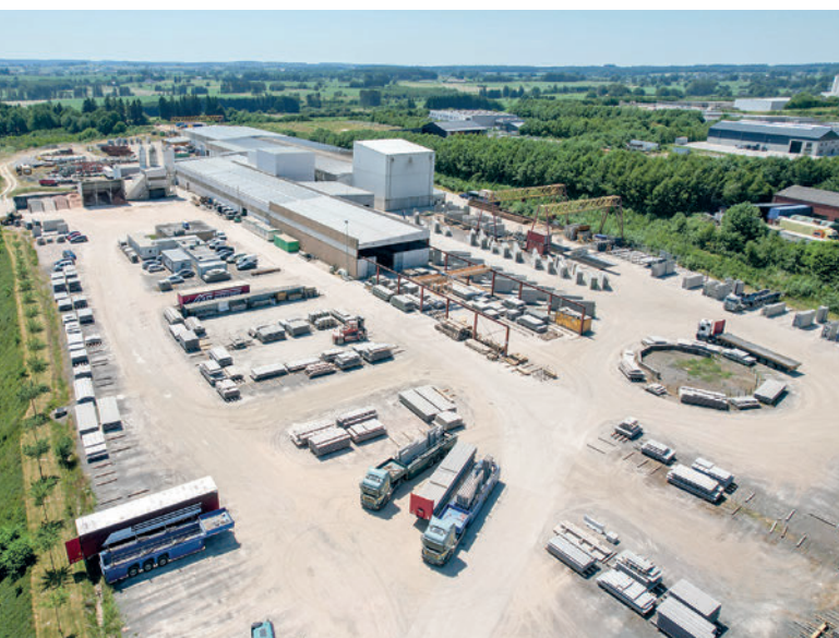
Alpha Beton has been producing precast concrete parts since the 1990s - initially with a lot of manual labour and now highly automated.
