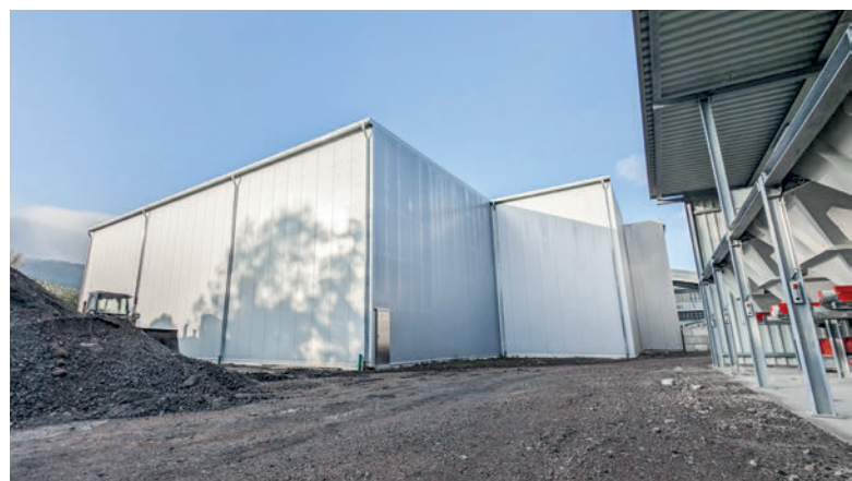
Curing chamber as a free-standing building and stainless steel escape door
