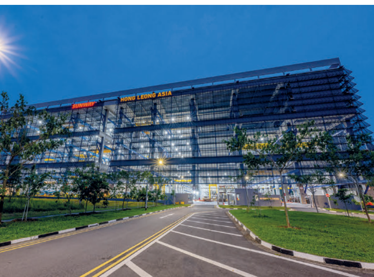
This enormous precast hub is the biggest of six planned to be built in Singapore over the next years.
