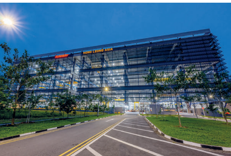
This enormous precast hub is the biggest of six planned to be built in Singapore over the next years.
