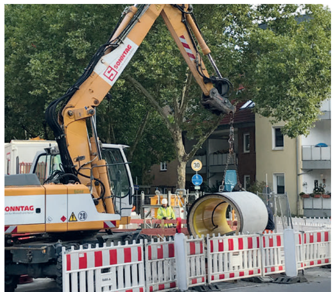
Datteln project: Lifting into the starting pit, piping detail with bentonite lubrication.
