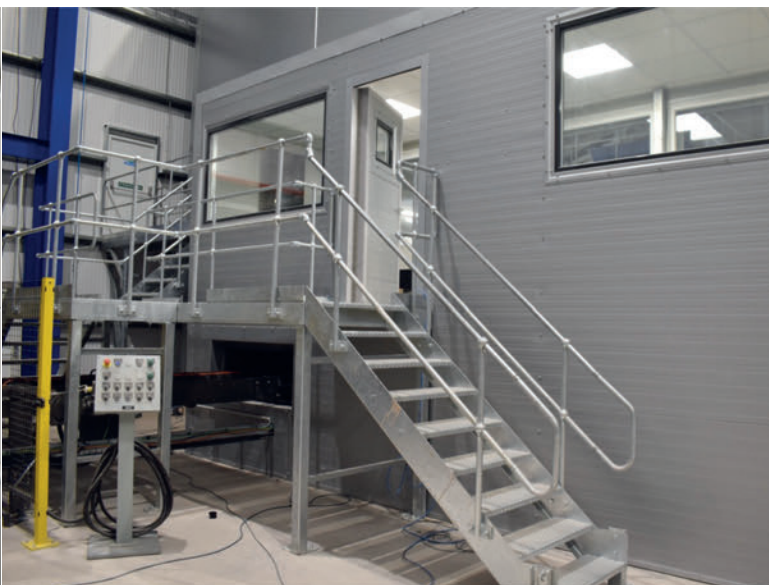
Unique window solutions allow for noise reduction and visibility into the factory and machine room.
