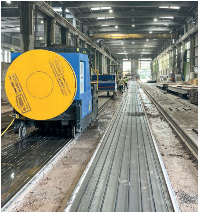
The hollow core elements are produced on 1.2 wide and ca. 150 m long beds.
