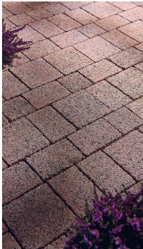
Bush hammered pavers with broken edges.
