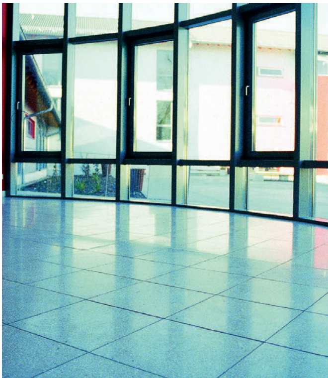
Ground slabs for indoor area
