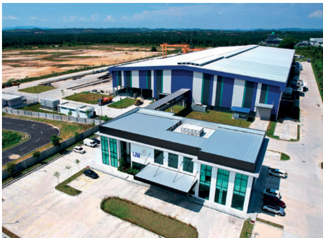
IJM IBS produces advanced precast products with Progress Group's automated machinery in Bestari Jaya, Selangor, Malaysia.
