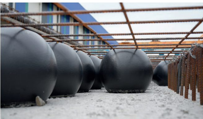
Innovative Bubbledeck slab system removes excess weight by using plastic bubbles as voids within the floor slab.
