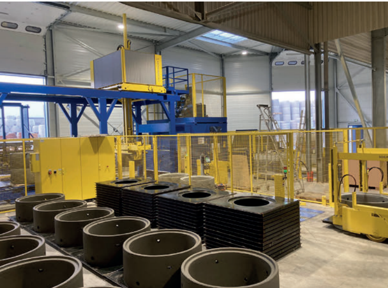
View of the palletizing system in the extension building.
