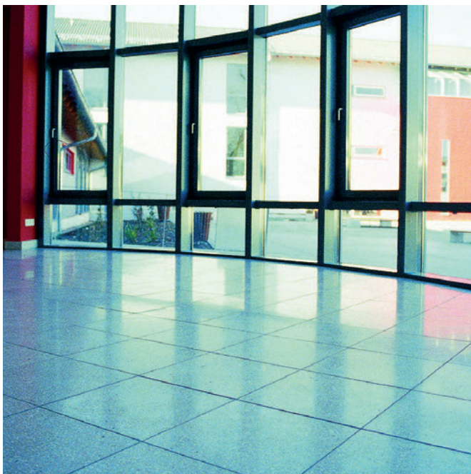
Ground slabs for indoor area
