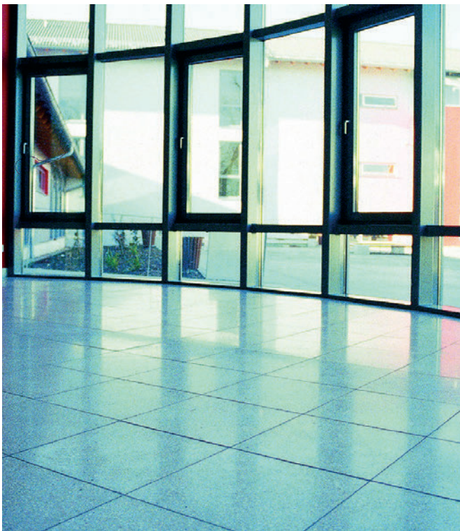
Ground slabs for indoor area
