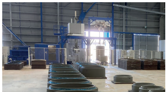
As well as the actual production, the palletizing of the products, and the cleaning and oiling of the pallets are all fully automated.
