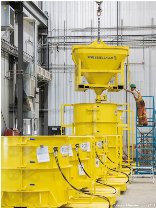
Moulds for different construction heights are filled with SCC.
