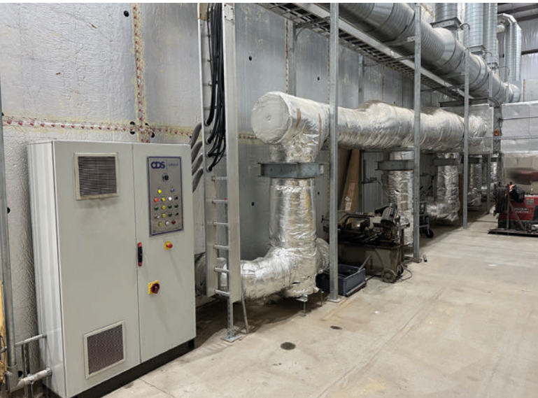
CDS Active Curing Chamber Environmental control maintains temperature and humidity.
