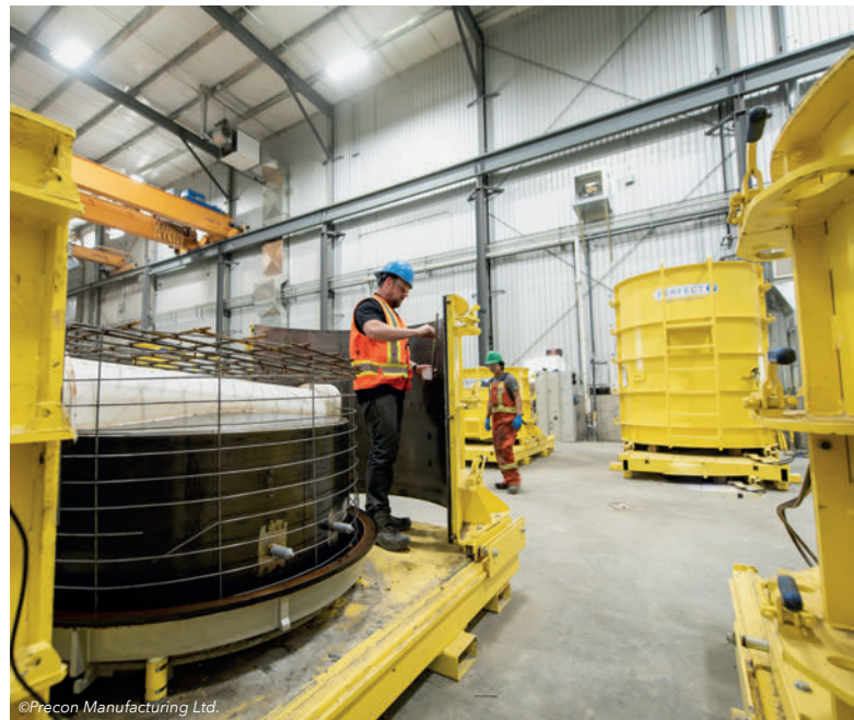
Setting up the channel, climbing aids, and reinforcement in the wall and floor.
