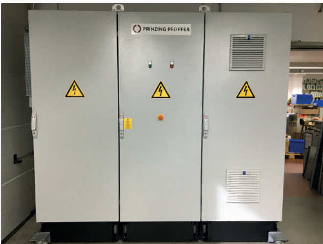
Electrical control system for the Radial Press RP 1230, built in a 3-door control cabinet including the latest worldwide proven Siemens Simatic S7 PLC technology
