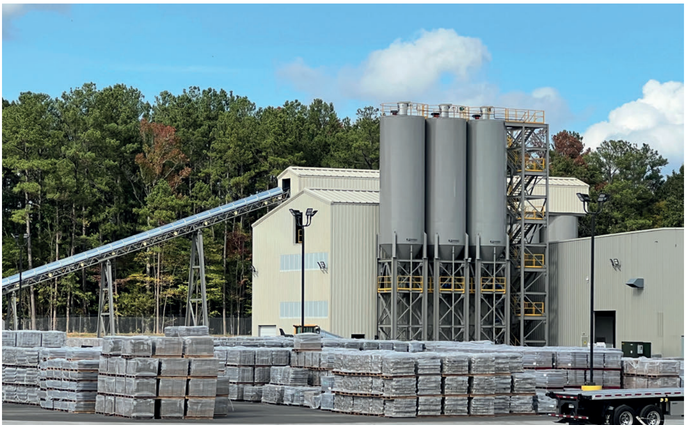
The new Oldcastle Adams Ridgeway plant is located just outside of Columbia, South Carolina and is producing high quality products in high outputs to service the regional market
