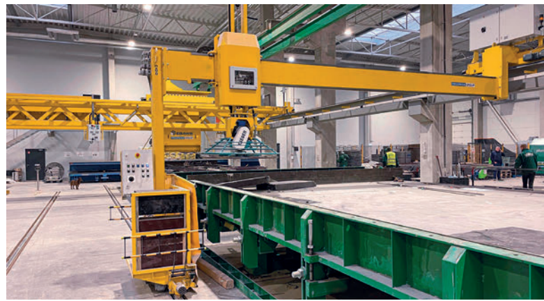
After the curing of the concrete surface the next phase is fine smoothing with a power trowel.
