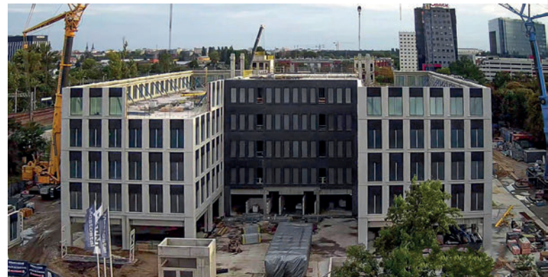
B10 office and hotel complex in Wroclaw (Poland).
