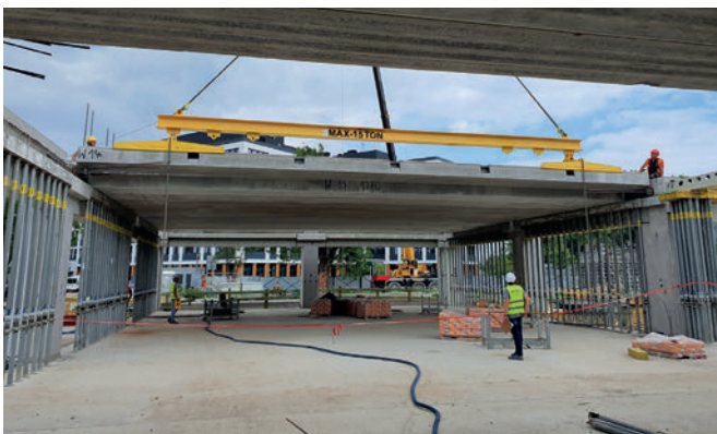
The prefabricated elements can be implemented faster and safer at the building sight.
