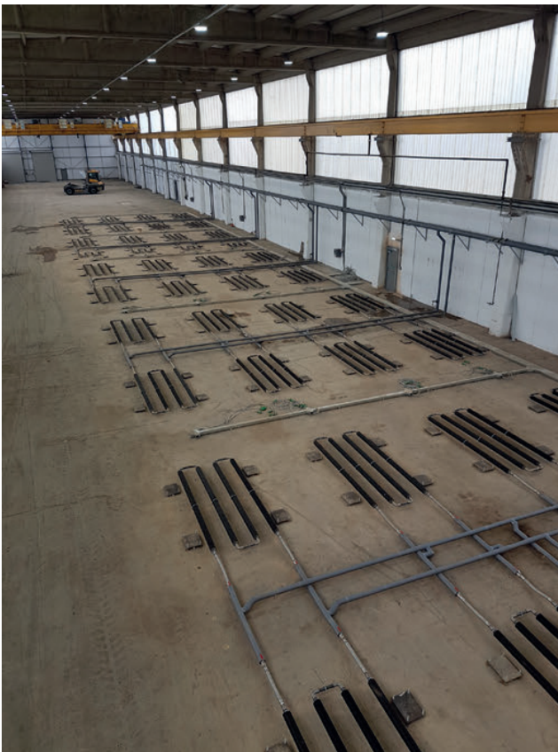
Heat distribution system designed by Kraft Curing
