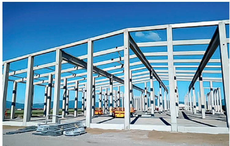
The beams and columns can be produced in the factory and then installed in no time at the construction site.
