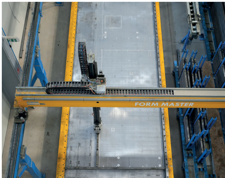
The shutters are placed exactly and automated according to the CAD planning.
