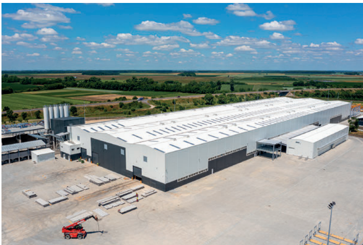
Viastein Kft belongs to the Bayer Construct group and is one of the biggest precast plants built in Hungary.
