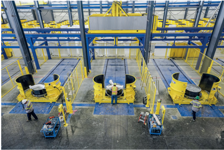
In all operating positions, value is placed on user-friendliness and efficient division of labor.
