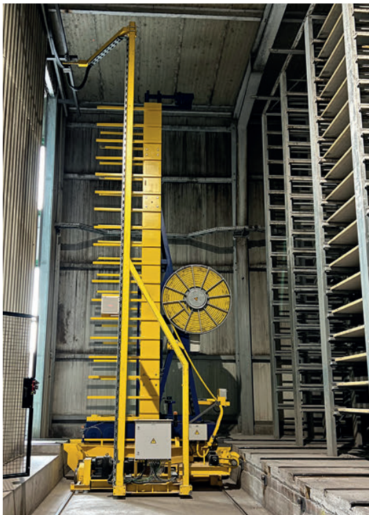
Finger car in the curing area
