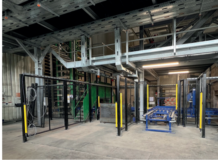
The wet side has now a station for safe discharge and quality control of the products
