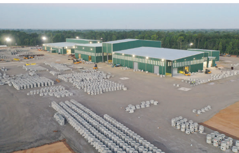
The first location of Ameritex Pipe & Products to be equipped with a highly automated wet cast production plant from Schlüsselbauer Technology in 2022.
