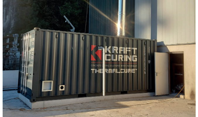
ThermalCure system made by Kraft is also in operation producing lining segments in Austria
