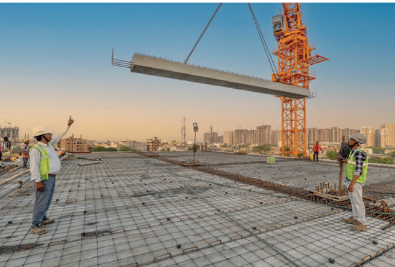
With prefabricated elements it takes significantly less time to build.
