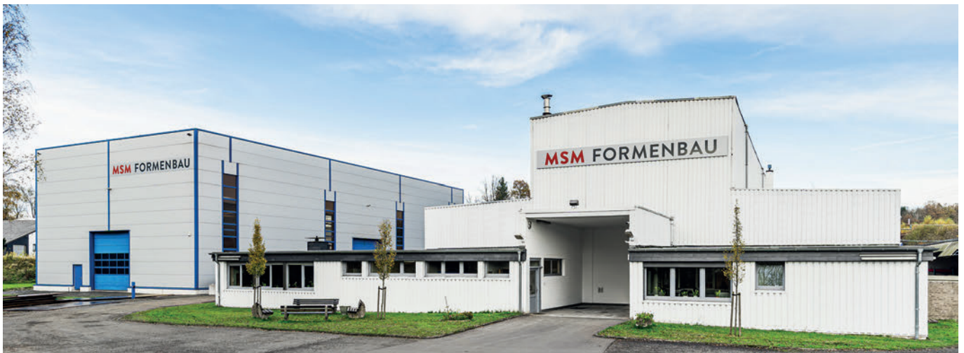
MSM Formenbau GmbH's site in Langenhahn with production halls and office building
