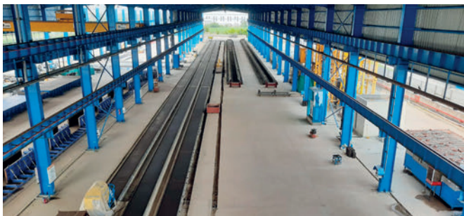
Overall four lines with a length of 145 meters are producing hollow core precast elements in the new plant of Stellar Precast.
