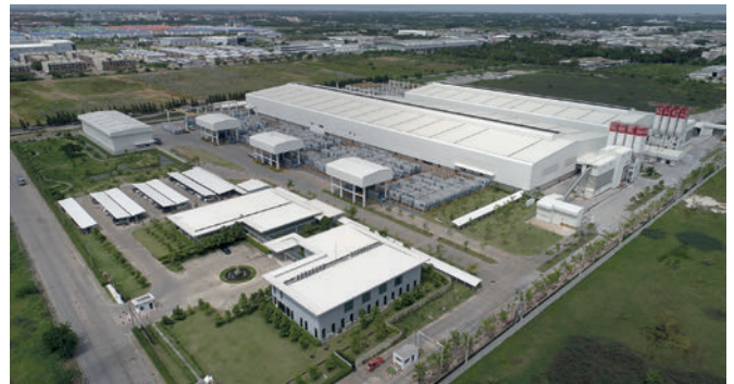
Pruksa was the first and is still the leading company investing in the production of precast concrete element production in Thailand.
