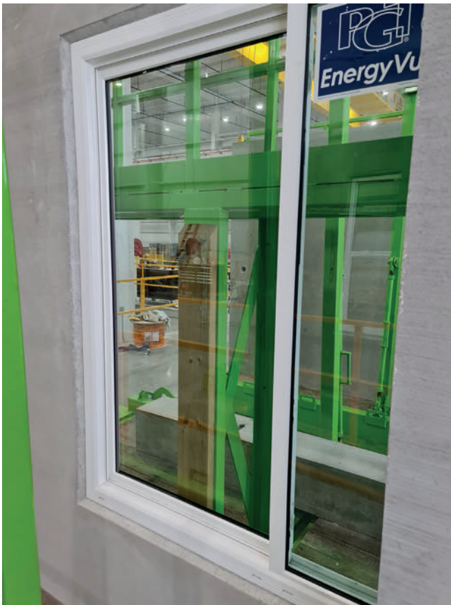
Completely cast-in windows – a special feature of the circulation plant
