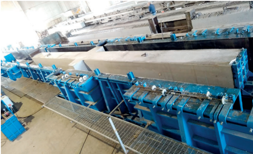
The produced pillars with corbels are 28, 5 meters long.
