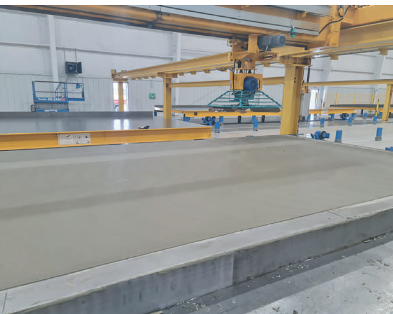
Three pallet lines are available for smoothing of the concrete surfaces.
