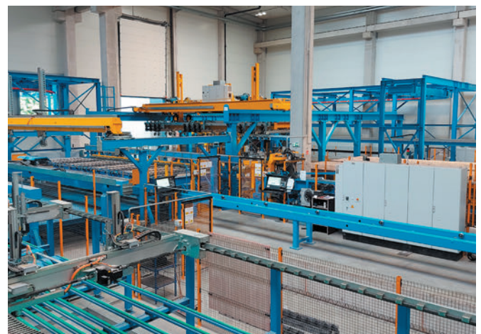
There are three production halls for precast walls, slabs and stairs.
