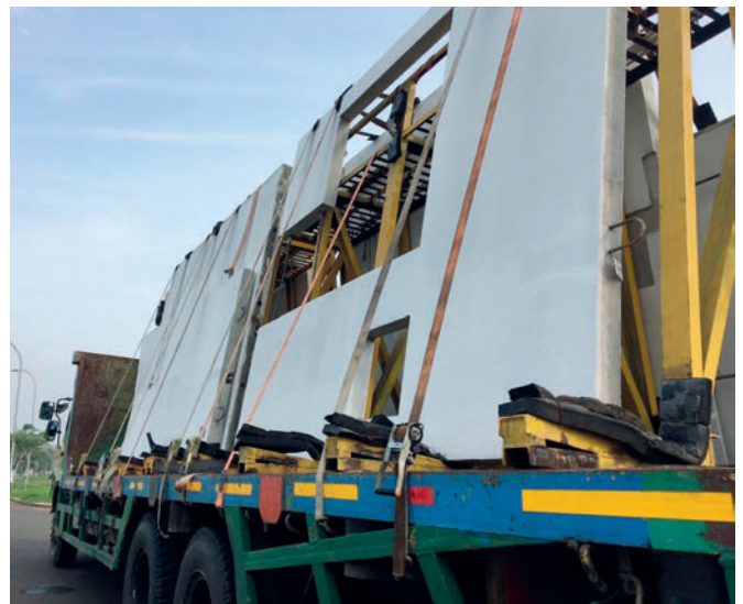
The earthquake tested and safe elements with the cut outs for doors and windows already implemented are transported to the sites.
