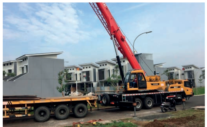
The building time is enormously reduced by building with prefabricated elements that are installed on site with cranes and qualified staff.
