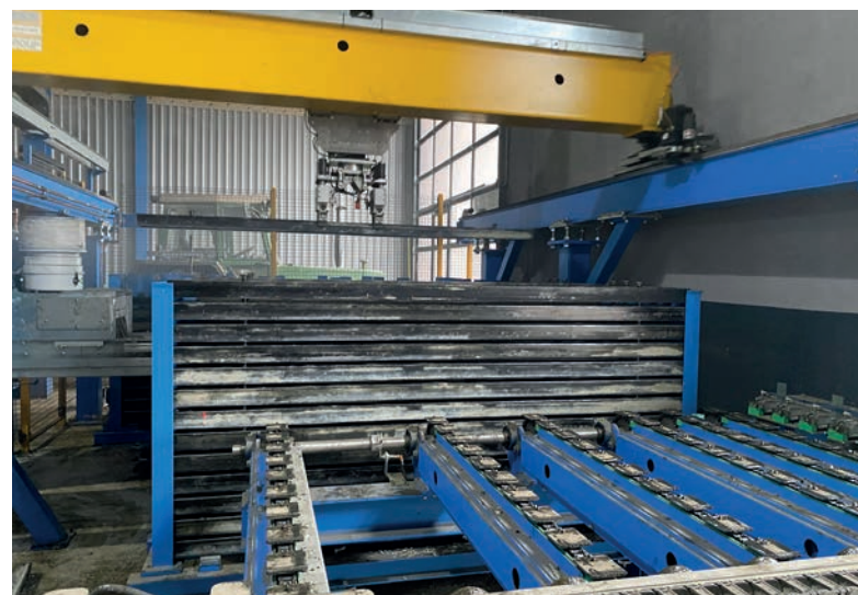
Storage robot in the active storage area
