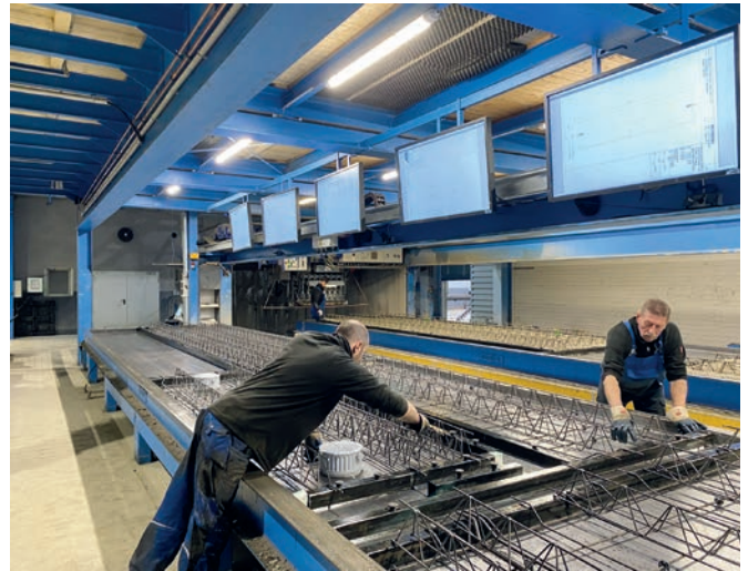
Final inspection of the reinforcement
