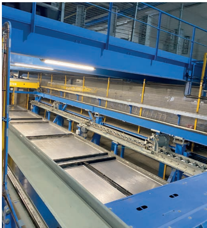
Form Master shuttering station
