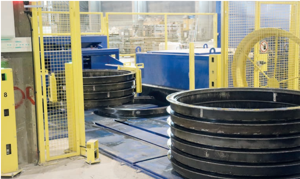
The cleaned and oiled pallets for subsequent use are stacked by the pallet stacking device
