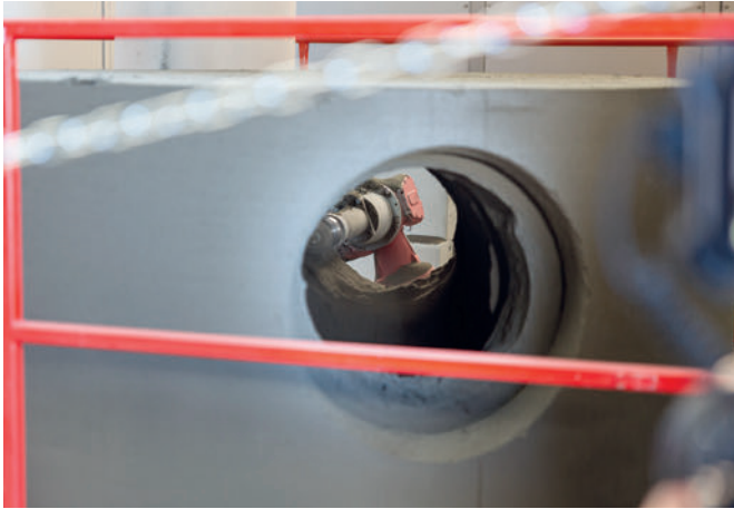
Concrete milling within millimetre accuracy with 2 different milling heads: for inlets and outlets on the left and for the channel on the right
