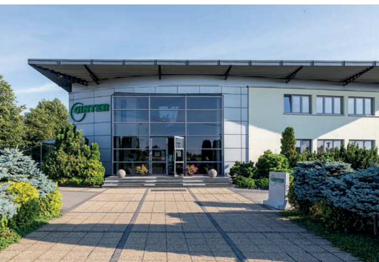
The headquarters of Ginter in Chojnice
