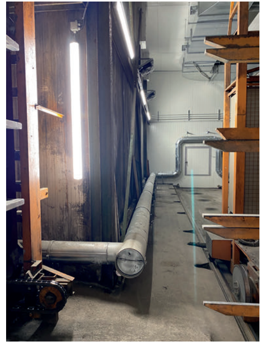
In the background you can see the insulated service door
