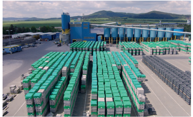
Production facility of Gebr. Ziegowski GmbH & Co. KG in Kruft, Germany
