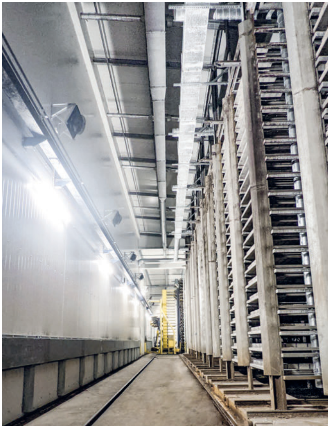
The transfer table aisle was also insulated; lights and fans were installed
