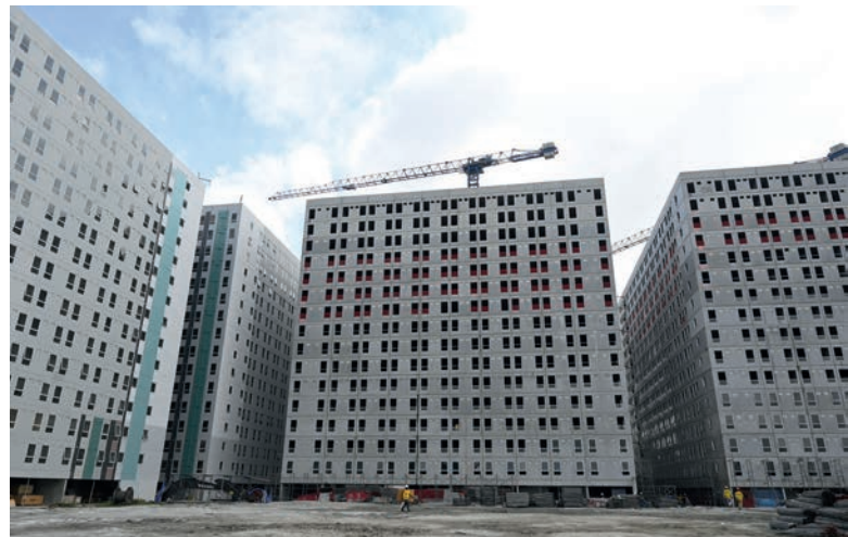
14-storey mid-rise affordable housing built with 90% precast
