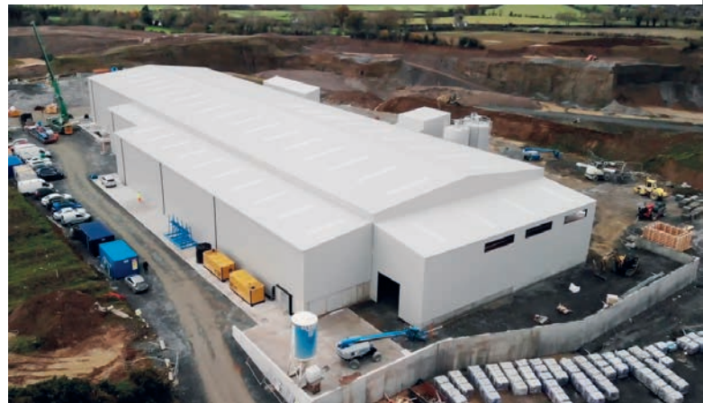
Kilsaran Precast in Kilcullen, County Kildare is the most modern and automated carousel plant in Ireland.
