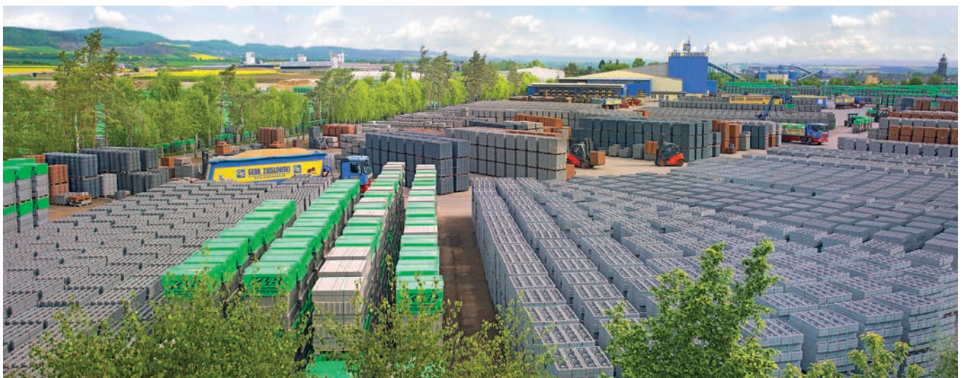
The efficiency of the Masa production plant is also reflected in the existing storage space (over 200,000 m 2 ).
