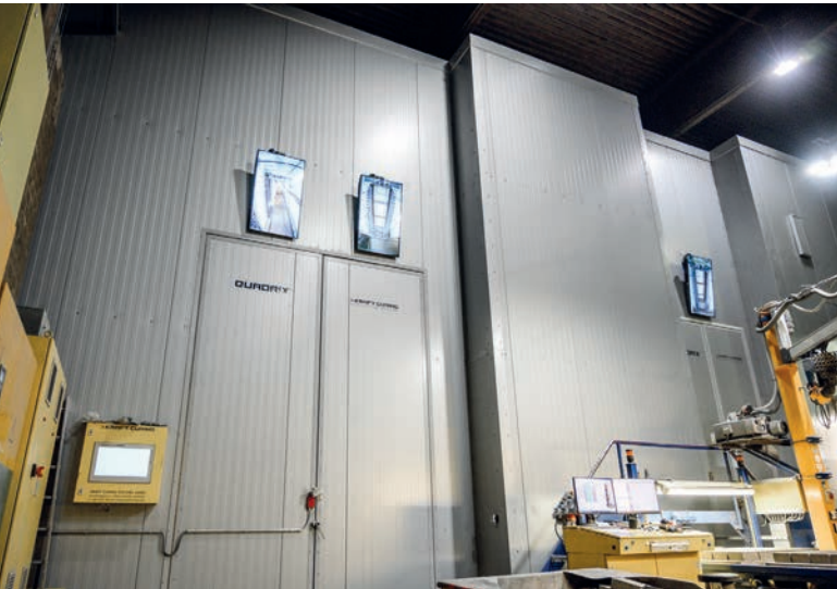
Elevators and lowerators are also completely enclosed in housing
