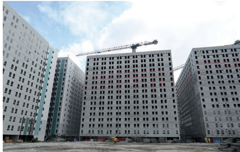
14-storey mid-rise affordable housing built with 90% precast
